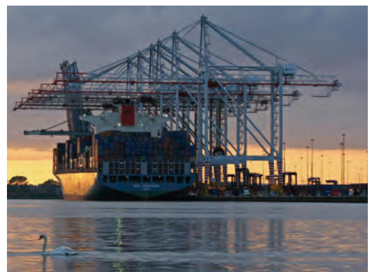
Ship to shore cranes.
