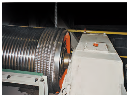
Hoisting mechanism in a steel picking line.
