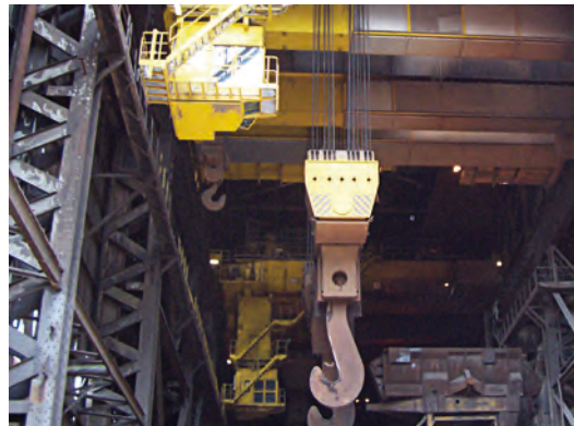
Travelling crane in steel mill.
