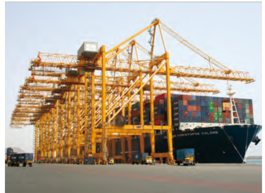
Ship to shore cranes.
