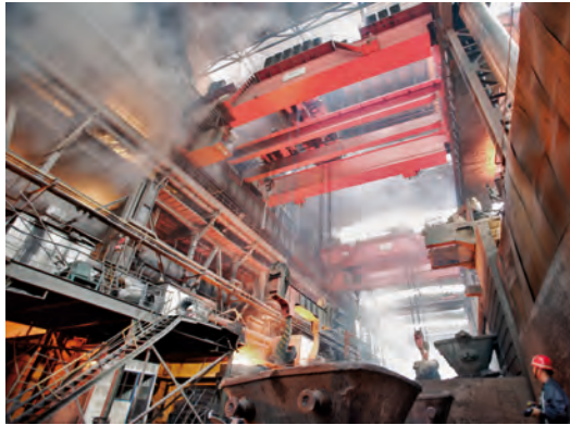
Travelling crane in steel plant.
