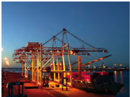
Ship to shore cranes.
